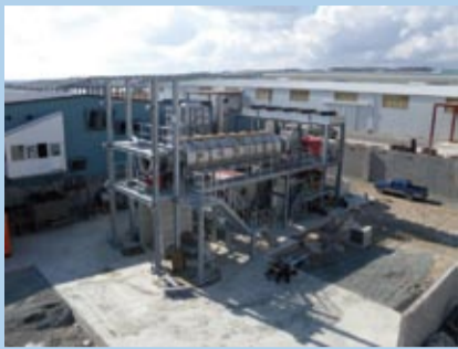
TechTrade Tyre Pyrolysis Plant in Cyprus
