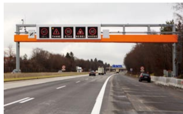
Overhead Displays at Motorway A2 Picture: Foto Peter Melbinger
